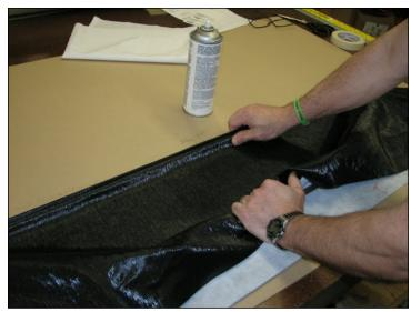
4. After the adhesive is "tacky", line up the binding along the front edge starting at the center. Work your way out pressing the cover into place keeping the binding lined up with the angle of the frame.
